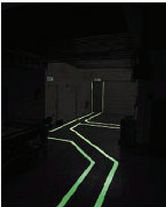
Figure 60: A 'way-guidance' system
