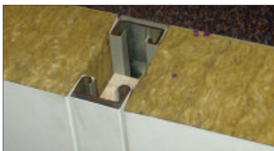
Figure 17: Insulated core panel – internal
