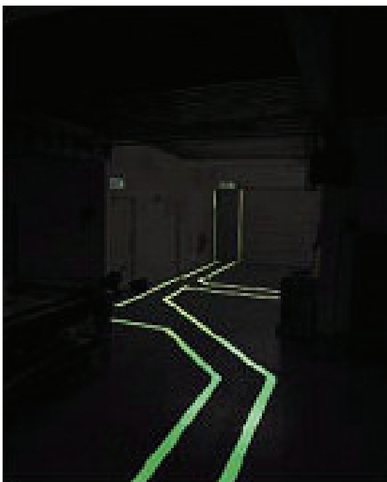
Figure 57: A 'way-guidance' system
