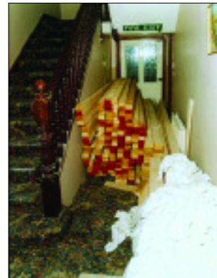
Figure 9: A blocked corridor with incorrect signage
