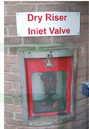
Image: Dry risers installed in a building to allow fire service to attach its hoses
