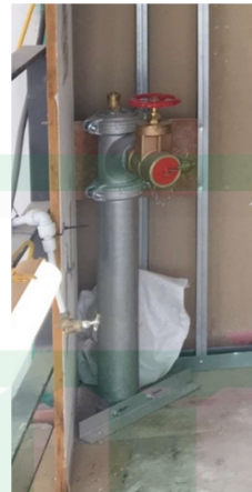
Image: Dry risers installed in a building to allow fire service to attach its hoses
