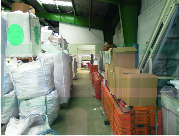
Combustibles on fire exit route
