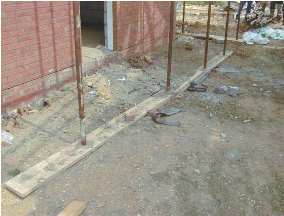
This image shows the standards and base plates on top of the Sole Board. If the floor surface is firm and level, the base plate may be erected straight on top of the floor surface.
